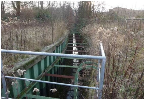
massiver Verbau: Spundwand
