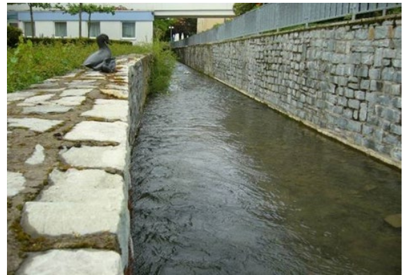
Technical standard profile (box-shaped)
