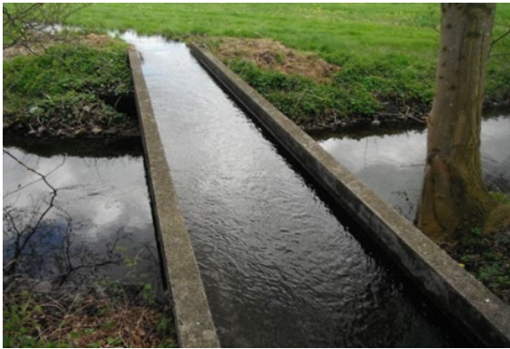
(Water)bridge, morphologically not harmful
