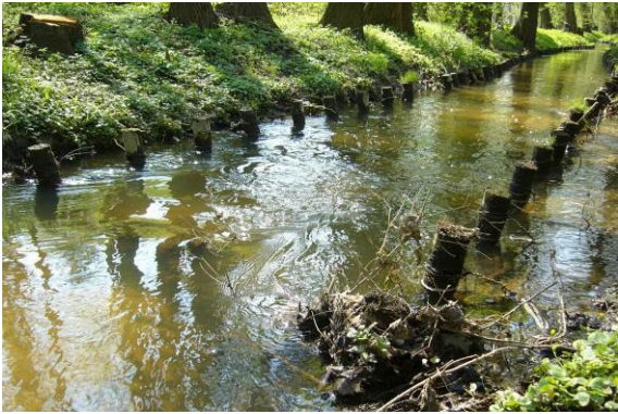
Technical standard profile, decaying
