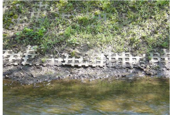
Massive bank protection: lattice blocks
