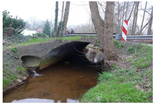
Culvert, natural embankment interrupted, with sediment
