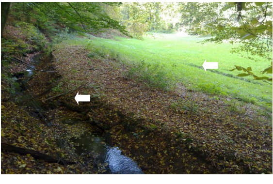
Relocation of the watercourse at the edge of the valley
