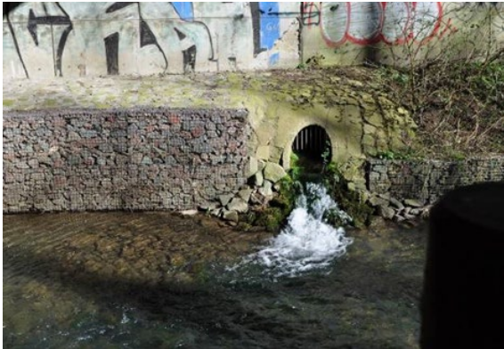
Massive bank protection: tile set, ungrouted (gabions)
