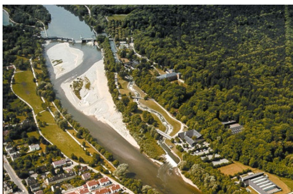
Movable weir >1 m with bypass watercourse (right)
