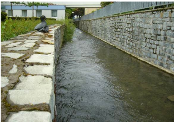
Massive bank protection: brickwork (grouted)
