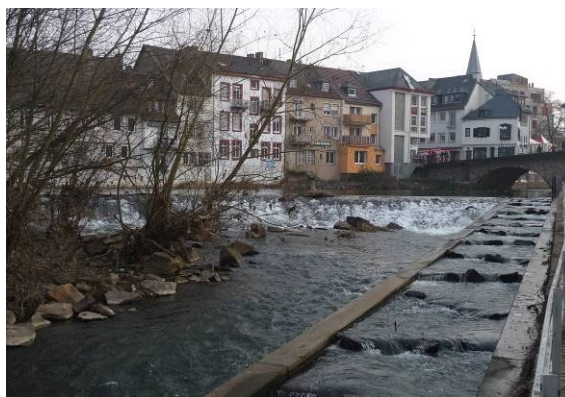
Bed fall >1 m with fish passage (fish ladder)
