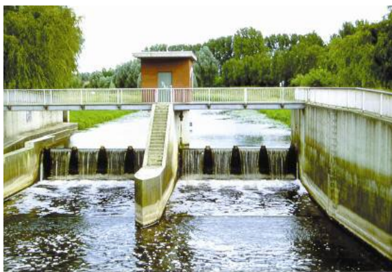
Movable weir >1 m with fish passage (left)
