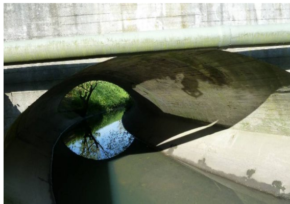
Piping/Overbuilding >10 m, without sediment
