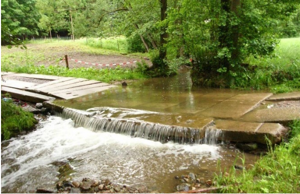
Solid bed substrate without sediment, <10 m (ford)
