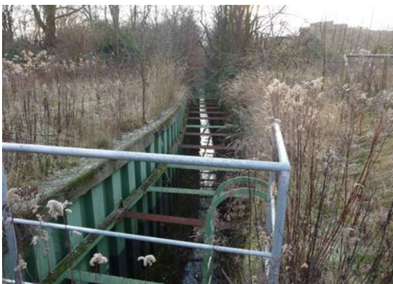
Massive bank protection: sheet pile wall
