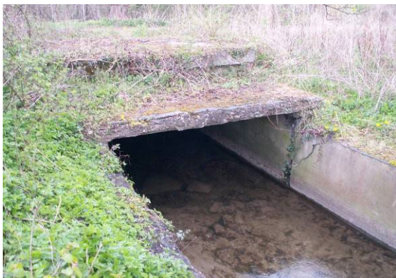
Piping/Overbuilding >10 m, with sediment
