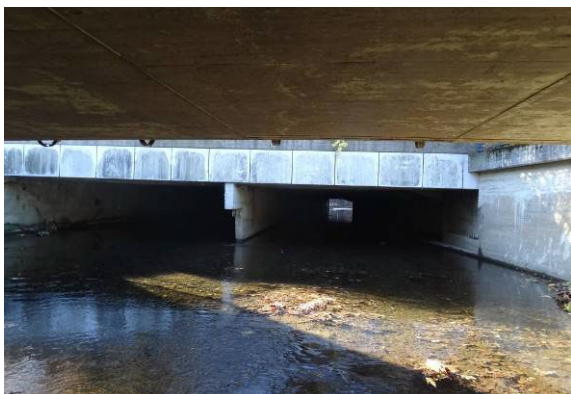
Piping/Overbuilding >100 m, with sediment
