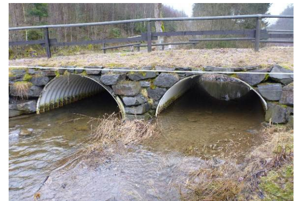
Culvert, watercourse narrowed, with sediment
