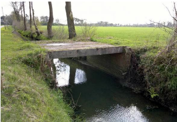
Bridge, natural embankment interrupted, with sediment
