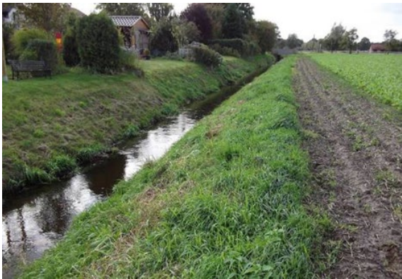
Technical standard profile (trapezoidal shaped)
