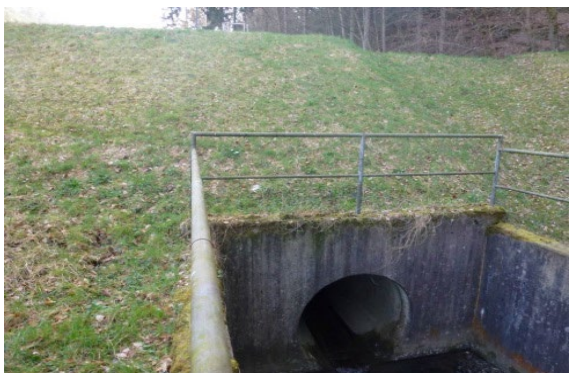
Piping/Overbuilding >10 m, without sediment (flow through an earth body of a flood control reservoir)
