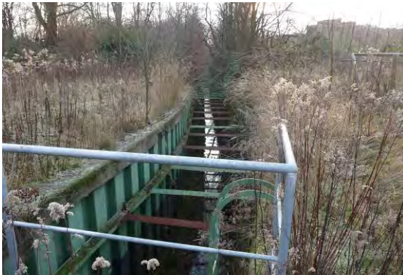
massiver Verbau: Spundwand
